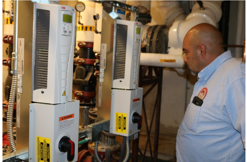
These new Variable Frequency Drives (VFDs) can be found in the mechanical rooms at Dane Smith Hall and were installed to improve the efficiency of the HVAC systems. Credit: Rachel Stone
