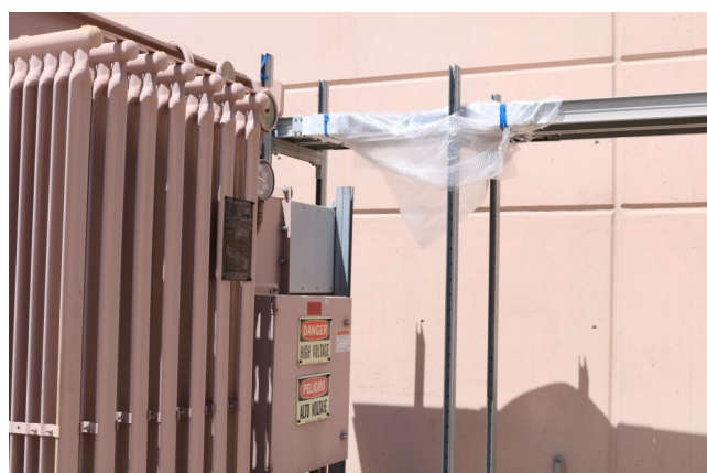
Technicians covered the damaged bus duct to protect from moisture until the repair can be completed. Credit: Rachel Stone
