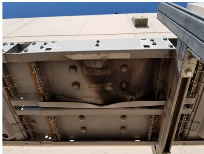
A view from underneath a damaged bus duct discovered by PPD Utilities technicians at the Lomas Chilled Water Plant. Courtesy of PPD Utilities
