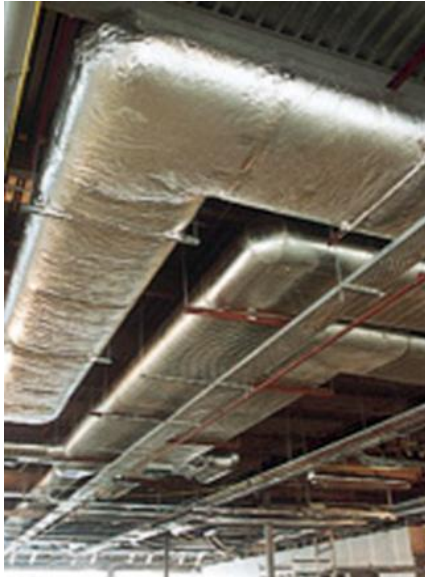
Typical HVAC Duct Work
