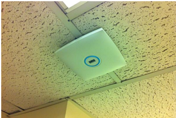
Typical Wireless AP at Ceiling.
