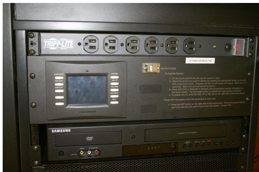
Crestron A/V Touch Pad System
