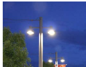
Full cut-off fixture only illuminate the area directly below.
